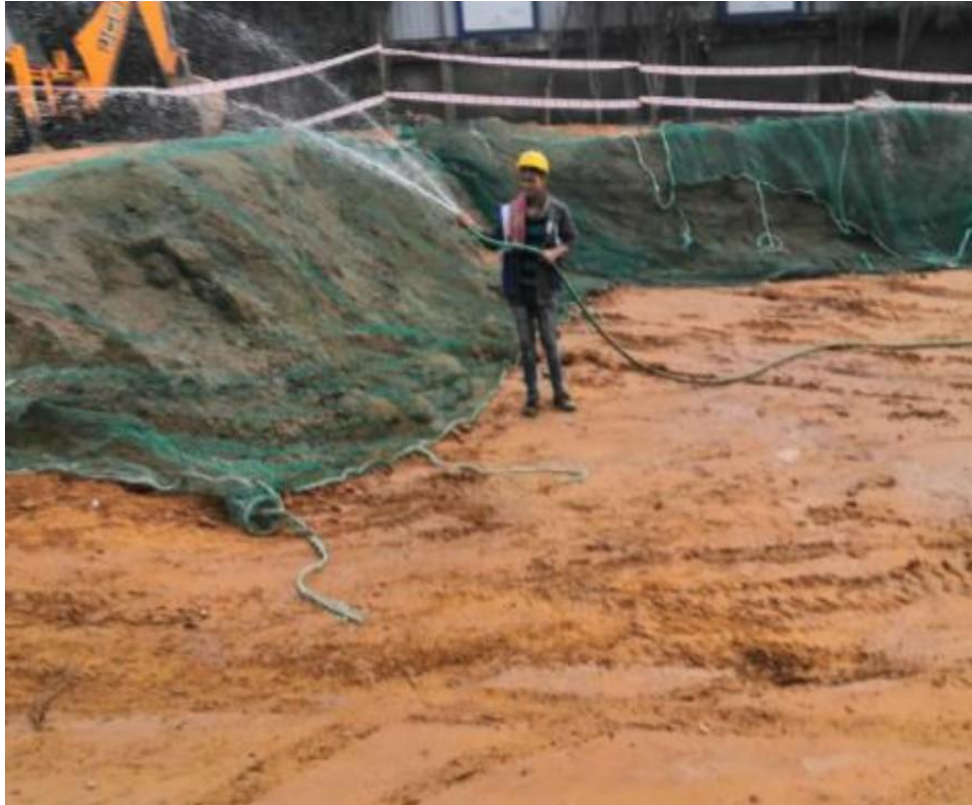
Photograph of Water Sprinkling at the construction Site
